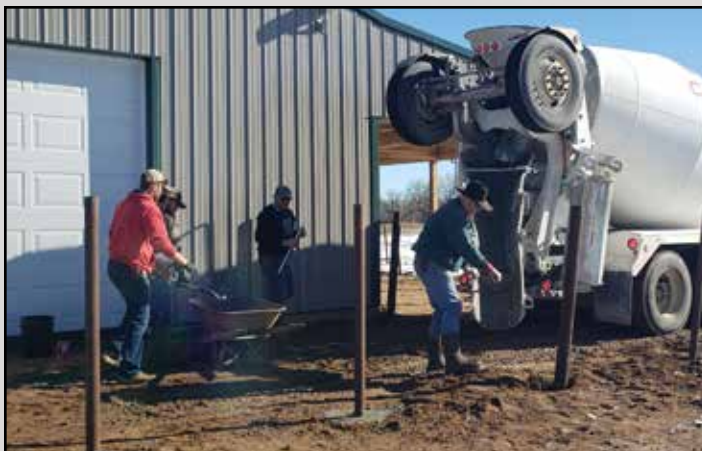
Constructing a new calving barn
